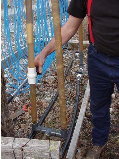
Figure 3. Opening Valve of Side by Side Two Pipe Sap Ladder with Valve
